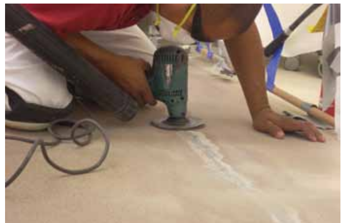
ABOVE ▲ “We used hand grinders equipped with 12” (30.48cm) disks to reach into the corners,” says Tabrizi. “We created a heavy profile.”
